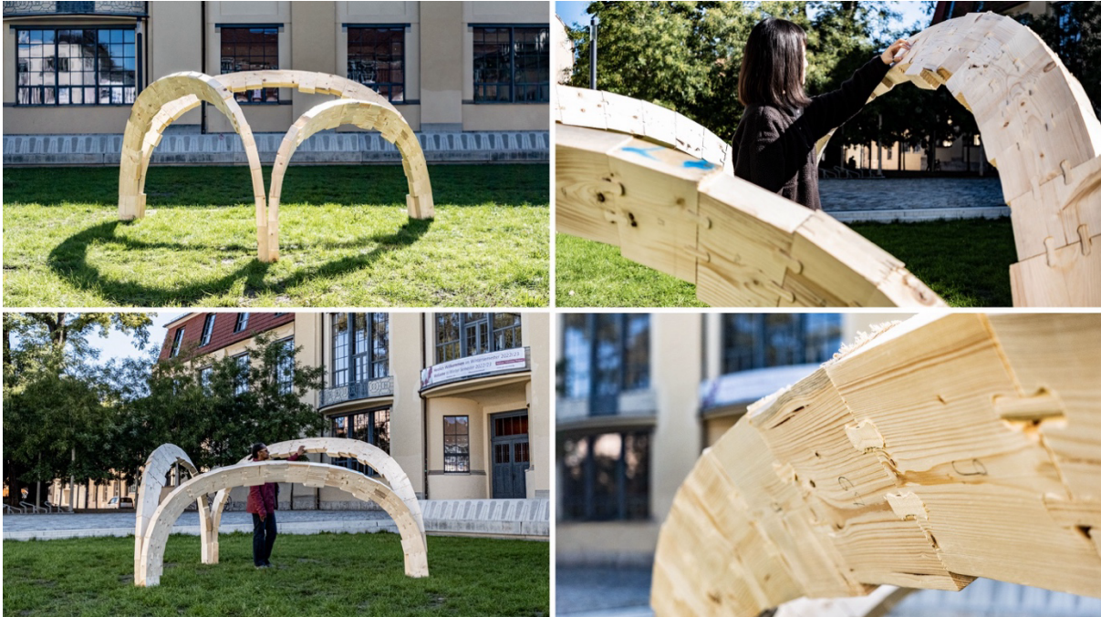
Figure 8. The Demonstrator, a Pavilion-Like Installation, Showcasing the Potential of Repurposing Offcuts for Free-Form Timber Structures. It Proves That the Conceived Computational Design Methods and Digital Fabrication Processes Are Suitable to Build Such Offcut Assemblies, Featuring a Unique Aesthetic Expression Driven by the Unprocessed Material. It Further Proves That These Digital Technologies Can Be Drivers for Circular Construction Practices. Photographs by Michael Braun, 2022.
