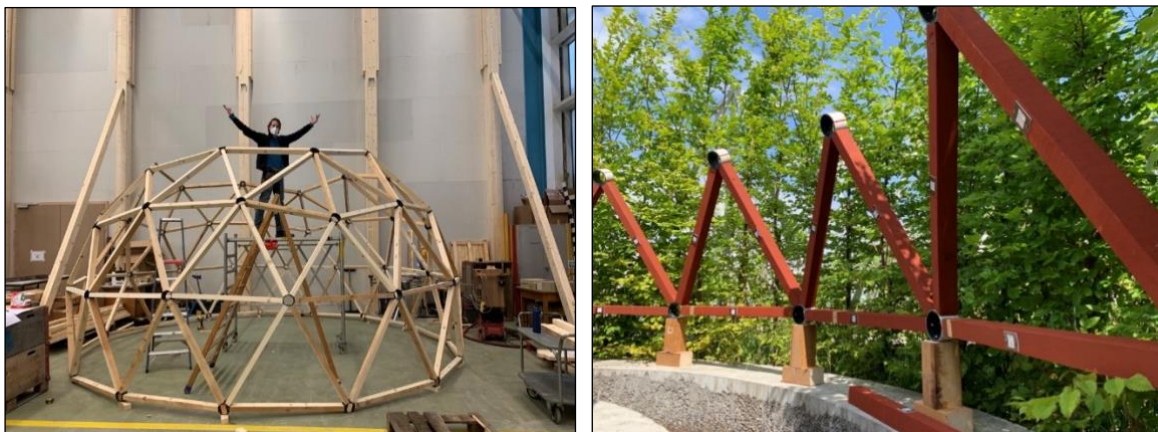
Figure 2. a) Construction of Dome1, and b) Construction of Dome2
